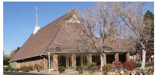
Sadly, 7 trees along the East side of the parking lot had to be removed due to the tripping hazards their roots were causing.
